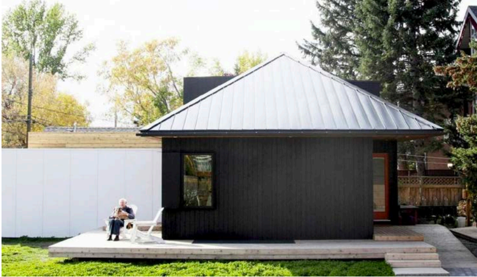
Figure 32: A Laneway house has been installed in the backyard in Calgary, Canada
